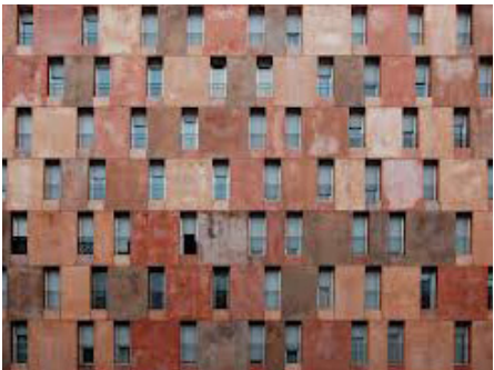
Rødlig beton, Madrid. Ark: David Chipperfield Architects
