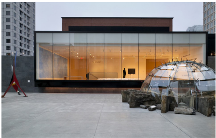
Oplyst top / prisme, MOMA San Francisco. Ark: Jensen Architects
