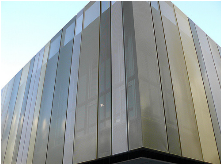
Transperant ydre facade, Bilbao. Ark: SENER
