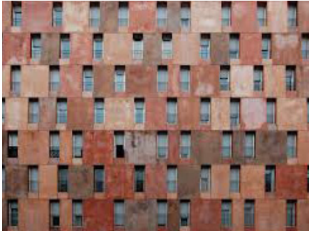
Rødlig beton, Madrid. Ark: David Chipperfield Architects
